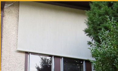
Shade moves with a solar motor operated from inside with a remote control.
